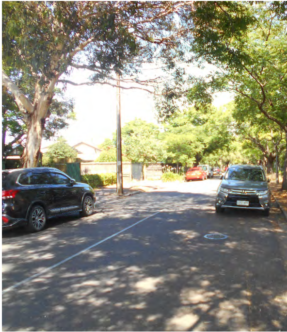
Figure 5: A 7-metre-wide carriageway and parking calms traffic on this residential street
