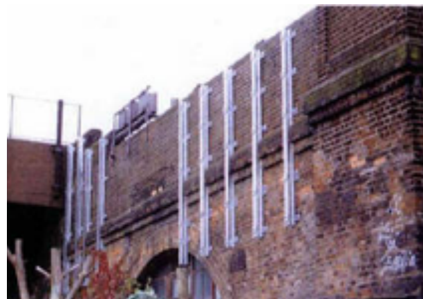
Parapet strengthening, Source: Cintec Canada, Thomas Network, 2011
