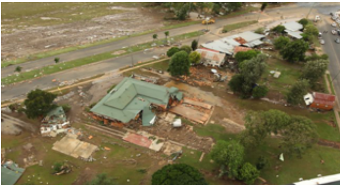
Damage to buildings in Grantham, Queensland, from 2011 floods
